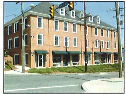
Stores separated from street by grade change
