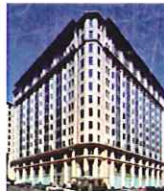
Office facade presents a beautiful corner.
