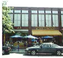
False second floor gives appropriate scale to one-story retail.
