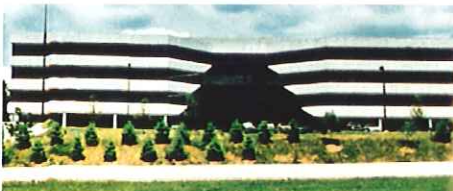
Building has no relationship to street; horizontal strip windows and cascading glass entry are inappropriate.
