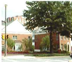
Lack of established corner defeats the feeling of spatial enclosure.
