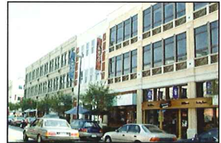
A long block can be broken into segments with changes in detailing and materials
