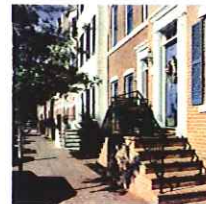
Streetscape is visually interesting for the pedestrian.
