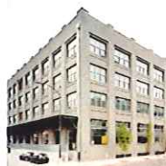
Building is a successful re-use for office/flex space.
