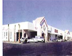
Successful re-use of an industrial building.
