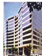
Concave facade interrupts pure street edge.
