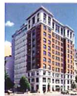
Punched windows and details at pedestrian level make streetscape.
