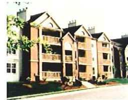
Balconies are so dominant they destroy sense of street.
