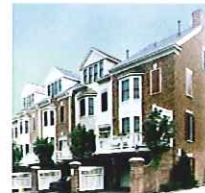
Rear garage is screened.
