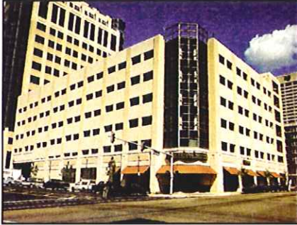
Parking structure with street-level retail
