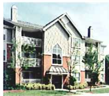
Under-scaled entry and tacked-on canopy have no relationship to the street.
