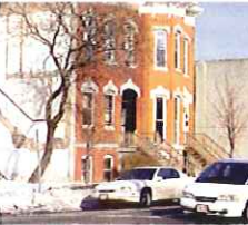
Empty house lot destroys street wall.
