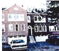
Entry stoops are too high above the street.
