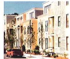
Variation in facade materials reduces the scale of large multifamily buildings.
