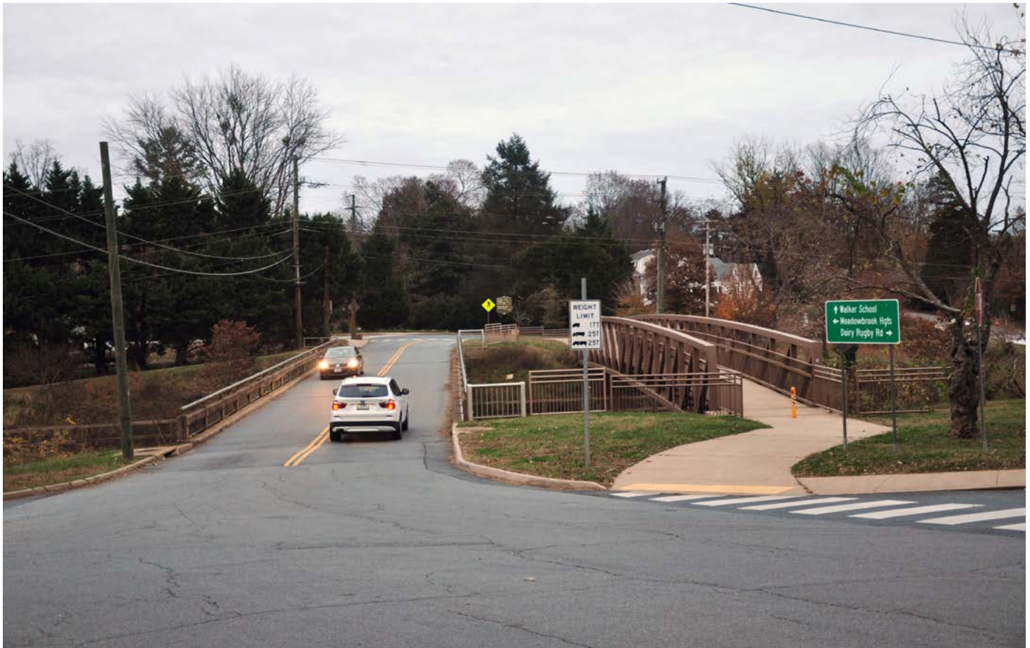
Preliminary engineering work continues on the locally administered project to replace the Dairy Road bridge over the U.S. 250 Bypass. To the right is the recently completed pedestrian bridge over the U.S. 250 Bypass.
