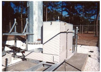
These two PCS equipment cabinets in Gainesville, Florida are smaller and lighter than cellular shelters. They do not need air conditioning. While less visible than facilities for cellular facilities, their visibility may be inappropriate in or near Avoidance Areas.
