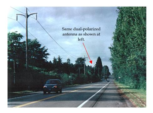
Installing a personal wireless service facility on a utility pole may require that the pole be changed from wood to steel. This photograph is from Clyde Hill, Washington, courtesy of Kirk Wines.
