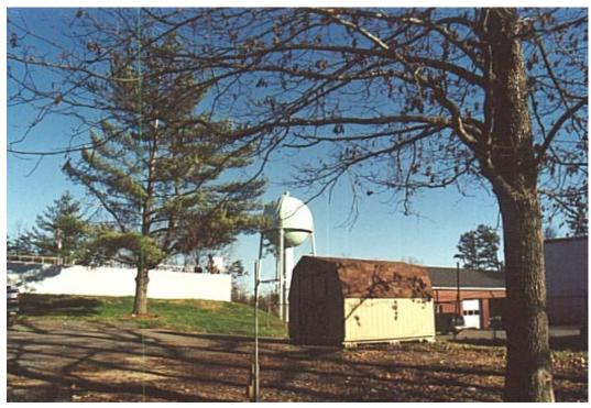
The Albemarle County Service Authority water tank in Crozet may be more suitable for side-mounted antennas rather than whips or panels placed on the top.
