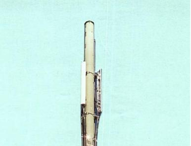
This antenna array on Barracks Road is sometimes called a "reindeer hat" or "top hat" array. These types of antennas can be found on transmission towers, lattice towers and monopoles.
