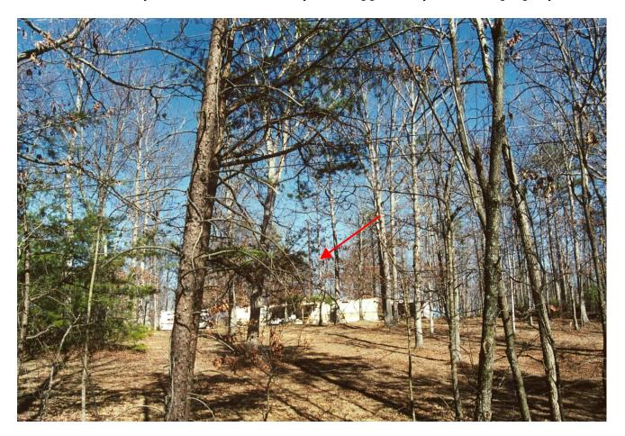
This monopole in Nix, although located on a high point of land, is virtually invisible because it is sited in the trees.
