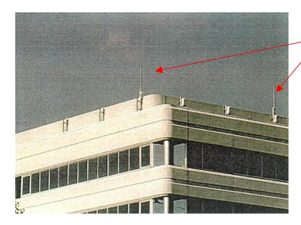
This photograph shows a conventional side-mounted personal wireless service facility on the parapet of an office building.
