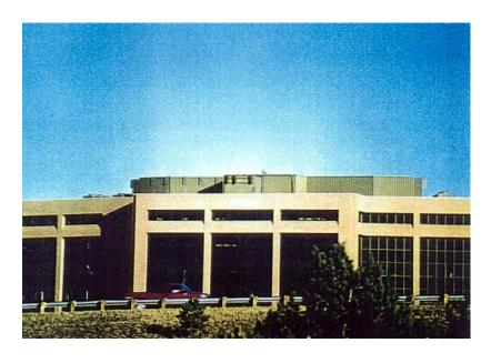
Roof-mounted facilities do not need to project up. They can be flush-mounted on the parapet or flush-mounted on a penthouse as shown on this office building in Arizona.
