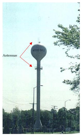
This co-location on a water tank in Illinois has antennas on the top and on the side. The side of the tank is better from a visibility perspective. (Photo courtesy of Specialty Constructors Coatings, Inc.)
