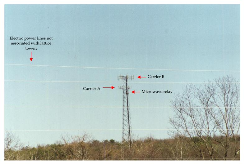
This is a tri-location of personal wireless service facilities near Boyd Tavern on a lattice tower. The microwave relay can be used for backhaul by both Cellular and PCS carriers, which also use wireline (telephone) for backhaul when it is readily available.
