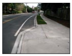
Figure 52 Bike lanes approaching roundabouts can have their own ramp onto the sidewalk, though most experienced riders will prefer to merge with the slow-moving traffic
