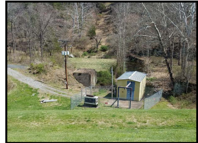
Existing Raw Water Pump Station 8
