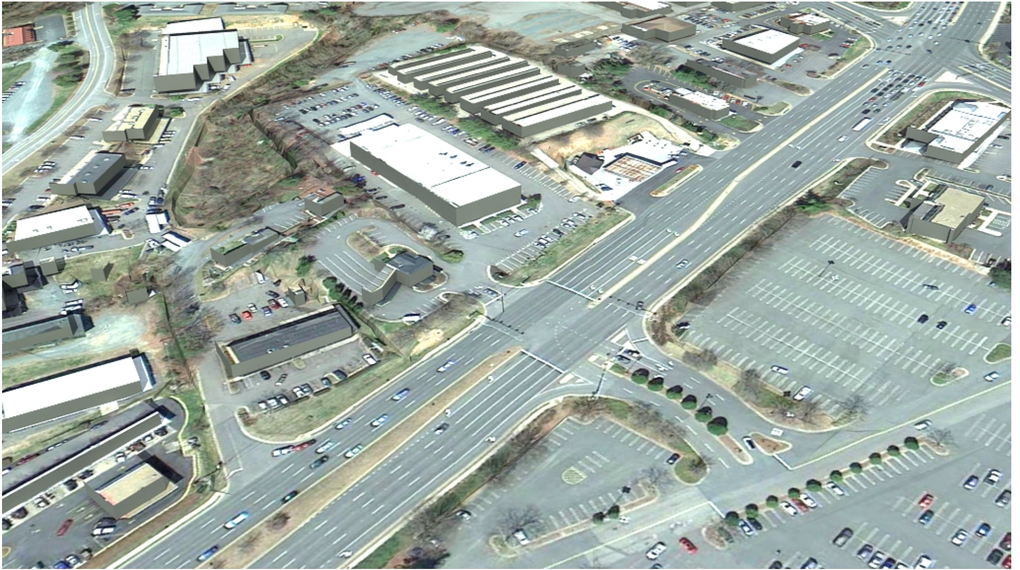
Existing approach to Rio Road Intersection
